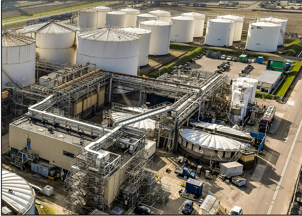
Figure 1.1: Example of petrochemical production unit and storage tanks
