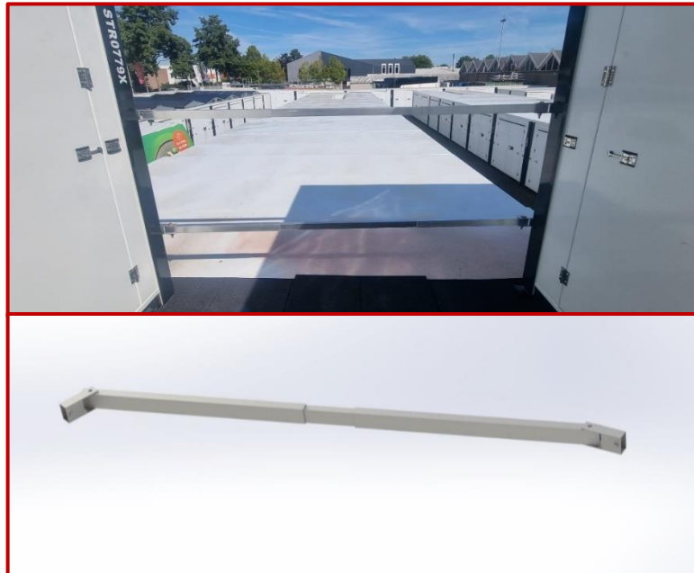
Figure 79 Railing installed in Deventer and its CAD counterpart
