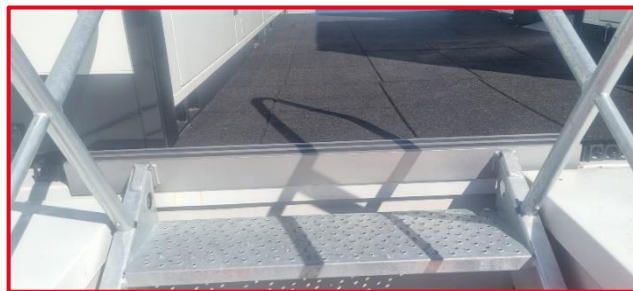
Figure 89 L-bracket for attaching the stairs
