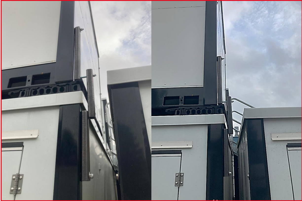
Figure 109 Bracket 5-2 test install
