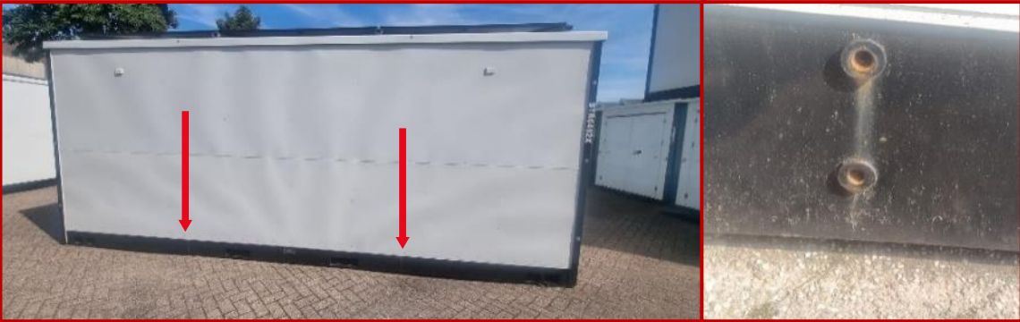
Figure 78 Mounting holes for the bridge
