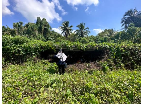
Figure 29. Uncontrolled vegetation on PV-panels
