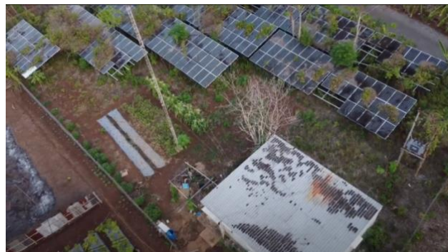
Figure 27. Overall view of PV Microgrid A
