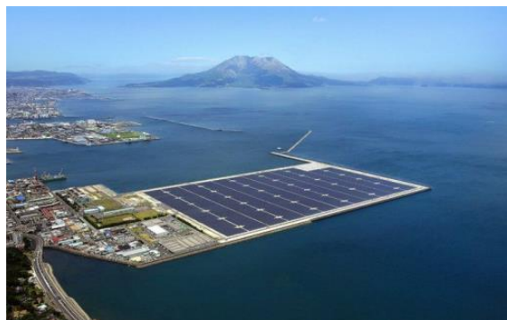
Figure 10: Floating PV microgrids (Ministry of Energy and Mineral Resources, 2020)
