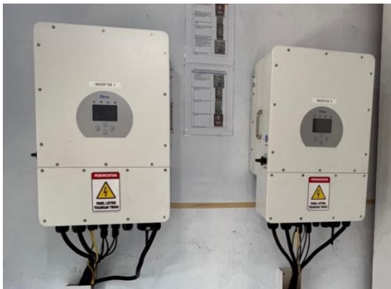
Figure 36. Hybrid Inverters
