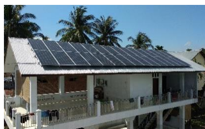
Figure 8: Rooftop PV microgrids (Ministry of Energy and Mineral Resources, 2020)
