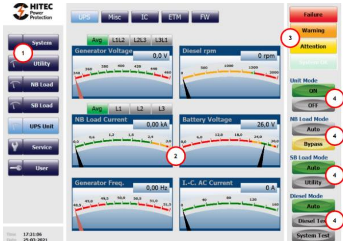
Figure 2.2: HMI panel layout of UCP for PP3600 (PP2700 can be found in Appendix A)
