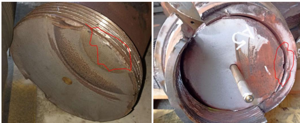
Figure 19, tie bar failures
