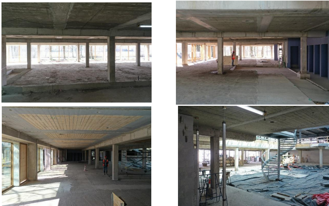
Figure 3.9. Construction Scenes of the New ITC Building (Source: Author)
