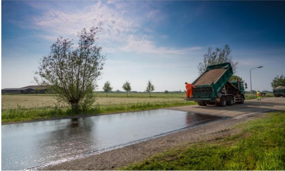
Figure 5. Application of single surface treatment (Crow, 2016).
