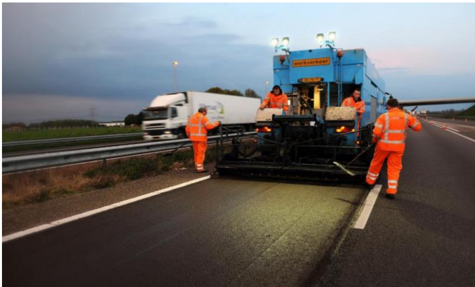
Figure 3. Applying ZOEAB (CROW, 2016).
