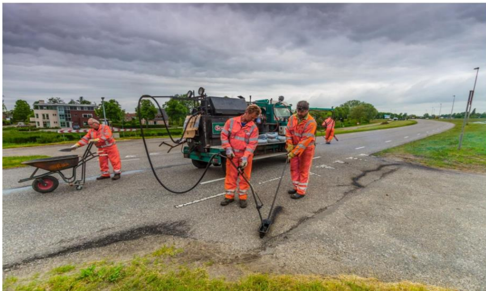
Figure 6. Crack filling (Crow, 2016).
