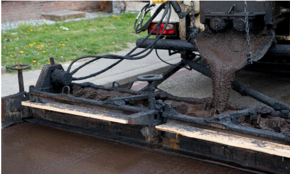
Figure 4. The application of EAB (Emulsie Asfaltbeton, n.d.)
