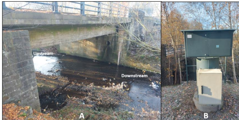
Figure 3.7. Location of the Measurement Station at the outlet of the Boven Geul Belgium near Kelmis. (A) shows the bridge under which the Boven Geul flows towards the Beneden Geul Belgium (The opening has a width of 12 meters and a height of 8 meters). (B) shows the measurement station. (photos: Jafeth Kuiper)
