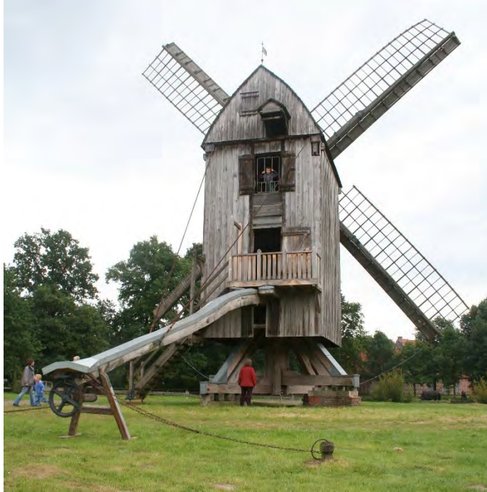
Figure 3 Post mill, rebuild in the open air museum Cloppenburg, Germany. The mill has presumably been build in 1683 at Essern, District of Nienburg Germany
