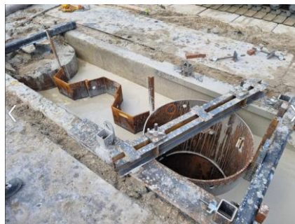
Figure 2: construction of cement-bentonite wall phase A Yangtze Canal
