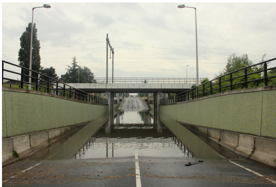
Fig. 13.1: Flooded viaduct in Enschede
