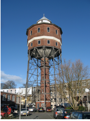
Fig. 3.2: An actual water tower [11]
