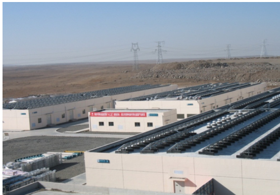
Figure 2.10: A storage facility in China (source: [67])
