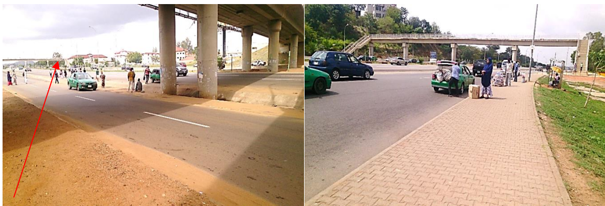
Figure 4-FF Views of pedestrian bridge at Banex junction
