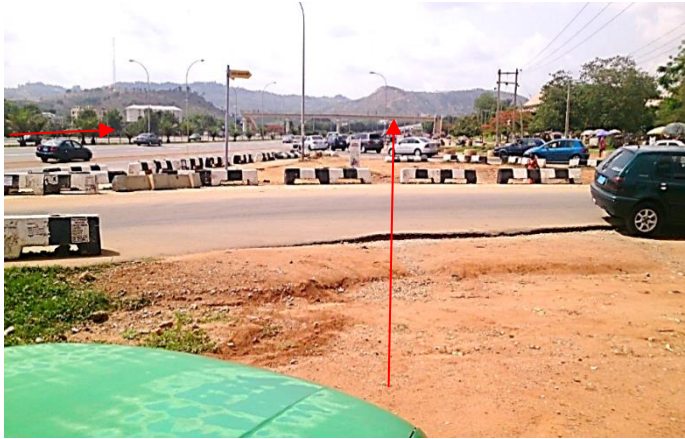
Figure 4-GG Pedestrian bridge and vandalised barriers at Nikon junction with obstructions Author (2018)
