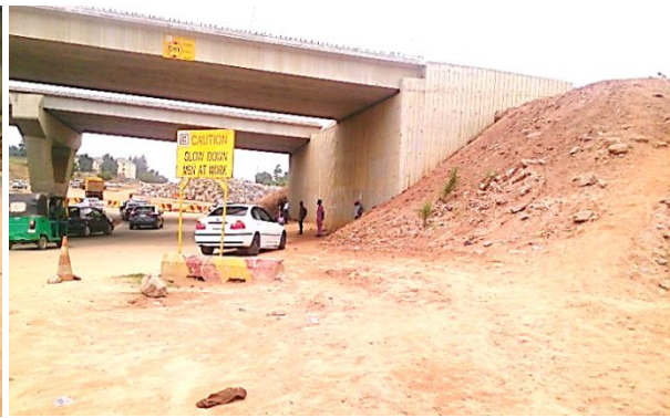
Construction work at roundabout
