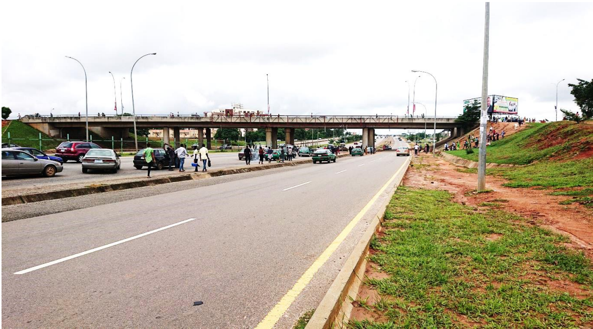
Figure 4-BB A view of Banex junction
