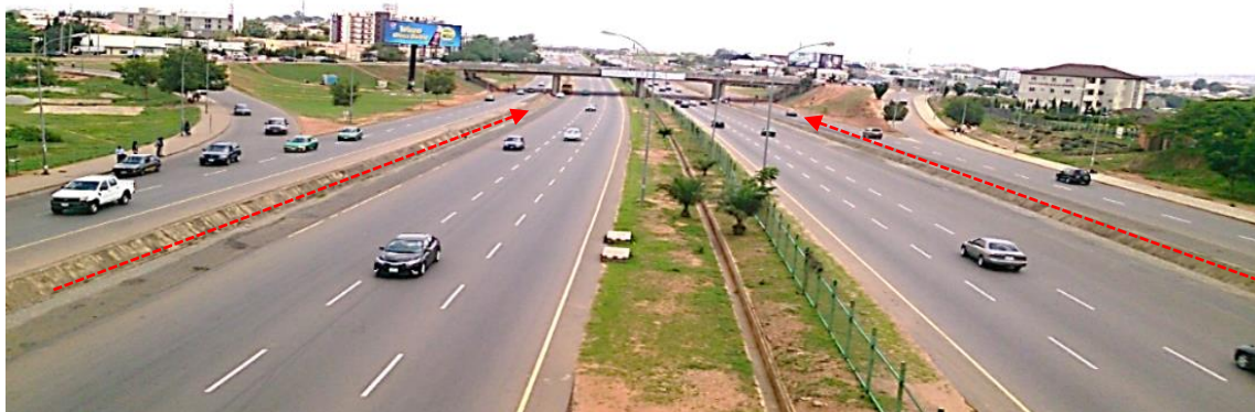
Figure 4-II Open drains in the middle of the roads
