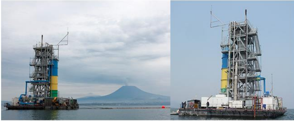
Figure 2.12 Pictures of the gas well in the Lake Kivu - from the Internet
