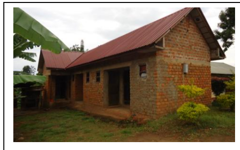
Figure 4-5: Photo showing house extensions done by land right holders
