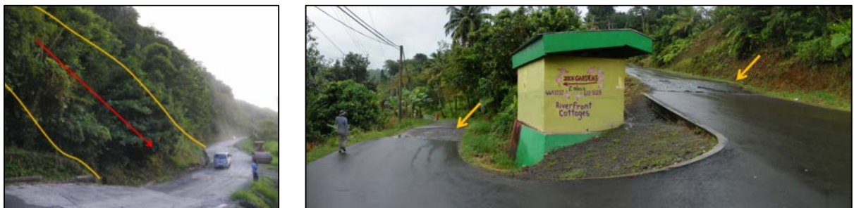
Figure 18. Landslides identified on fieldwork in Dominica. Deux Branch Area (Left), and Belle Wet Area Junction (Right).
