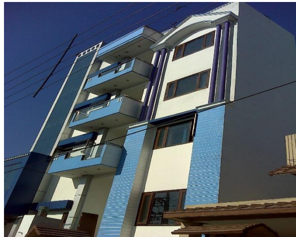
Figure 4-8 : Building type RC1M of ward no.33 on ground
