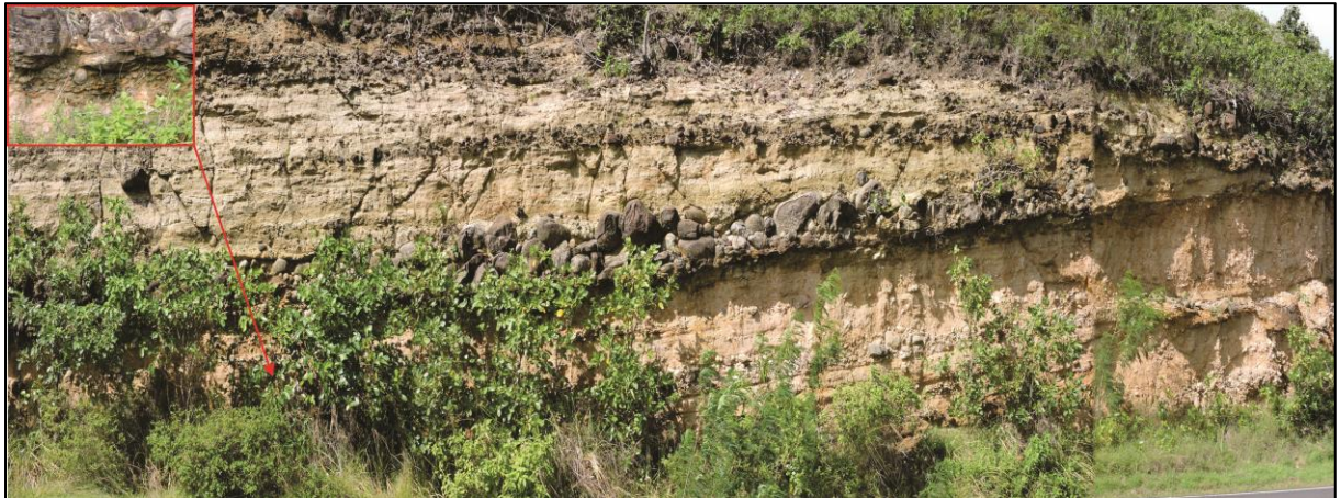
Figure 44: Cut slope L4
