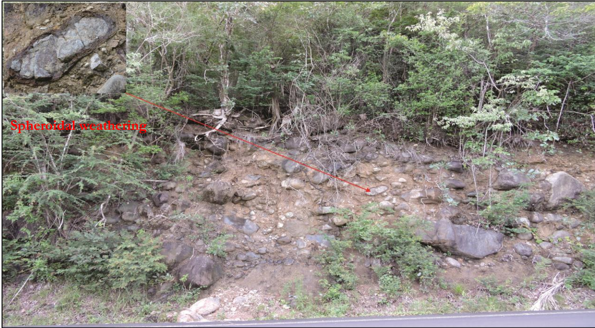
Figure 51: Cut slope L11
