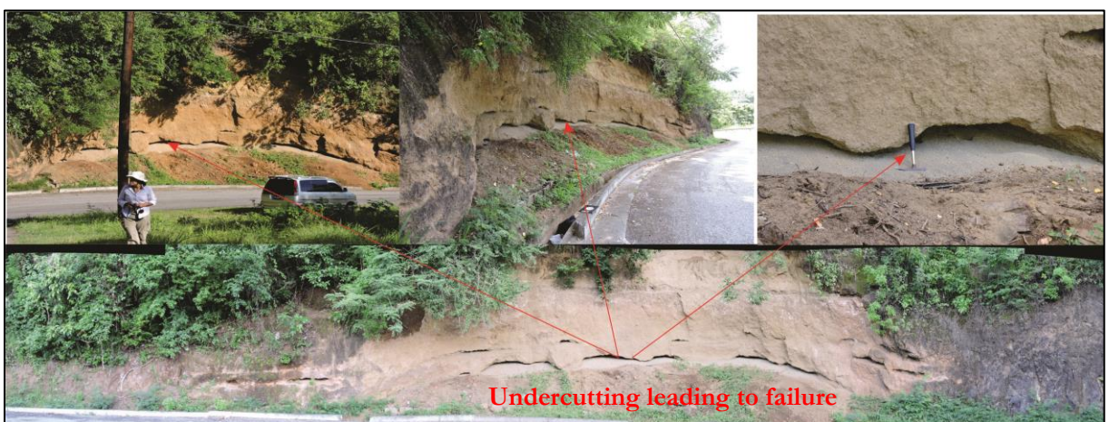
Figure 40: Cut slope V3
