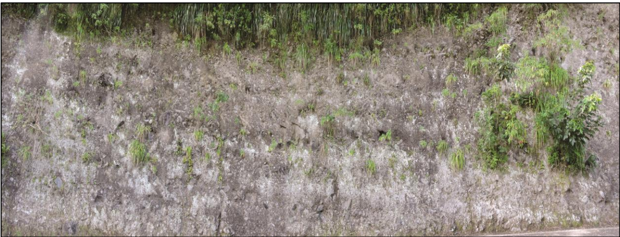
Figure 47: Cut slope L7
