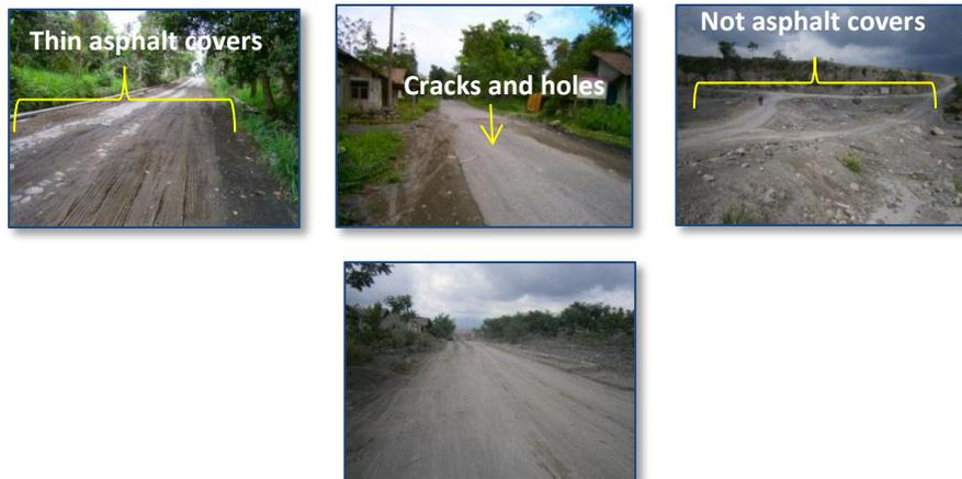
Figure 5-2. Damaged road caused by truck (1) Damaged road caused by lahars crossing Gendol river (2) (left side) and damaged road caused by lahars (3) (right side)
