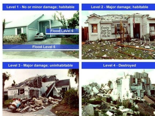
Figure 15. Damage assessment from photograph (Broward, n.d.)
