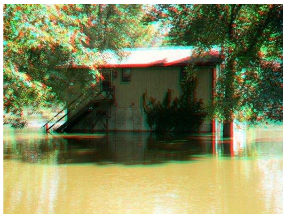
Figure 8. Anaglyph 3D Photograph of flooded house (Fototing, 2007)
