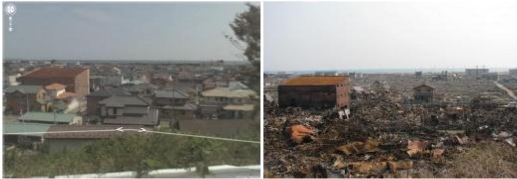
Figure 6. Disaster damage seen from geotagged photograph (Fontugne et al, 2011)
