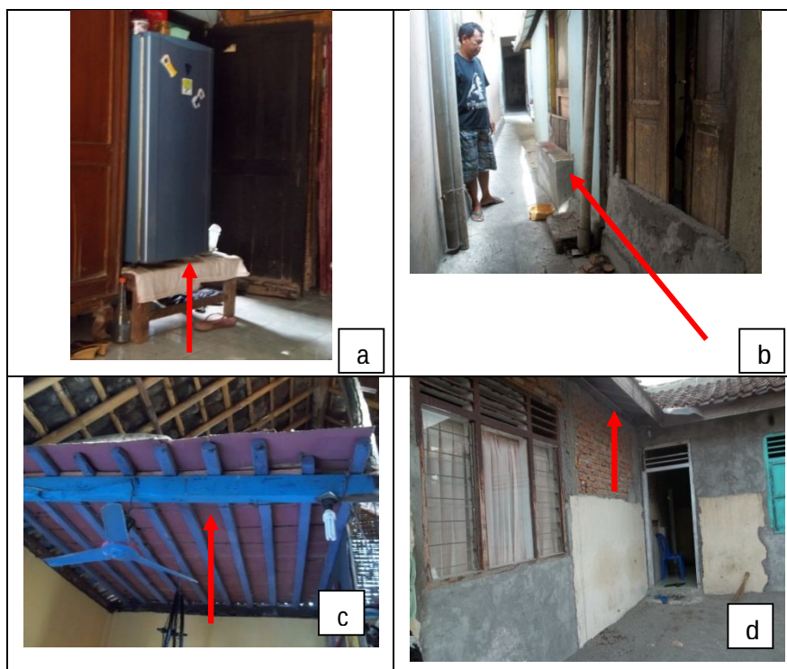
Figure 6-1. Households' coping mechanism. a). Move house property and valuable things in the higher place, b). Build door protection from concrete materials, c). Build a ceiling platform to store valuable properties and food, d). Raising the house. Source: Fieldwork (2011).
