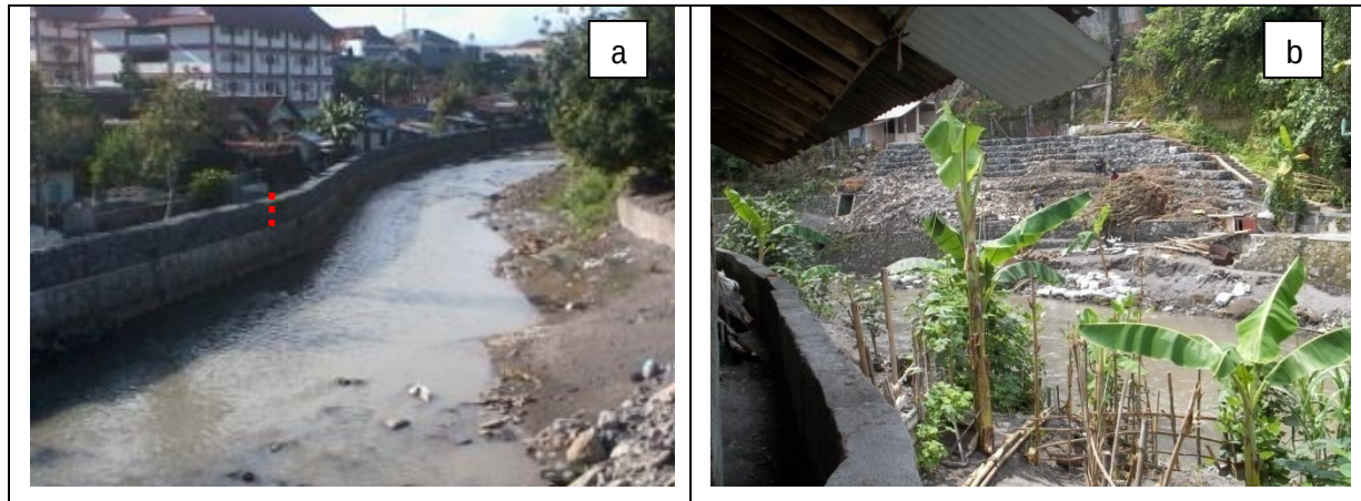
Figure 6-4. a). Raising the dike at Gowongan Subdistrict, b). Strenghtening the river embankment at Terban Subdistrict
