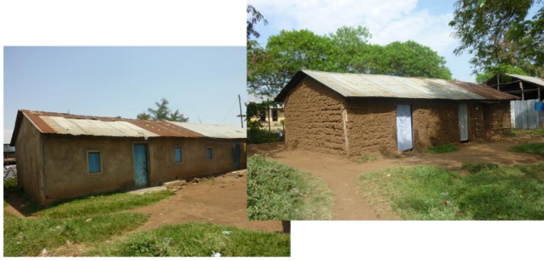
Figure 6-1 Photograph showing spectral differences in a single roof. It also shows the similarity of roofs and bare land.
