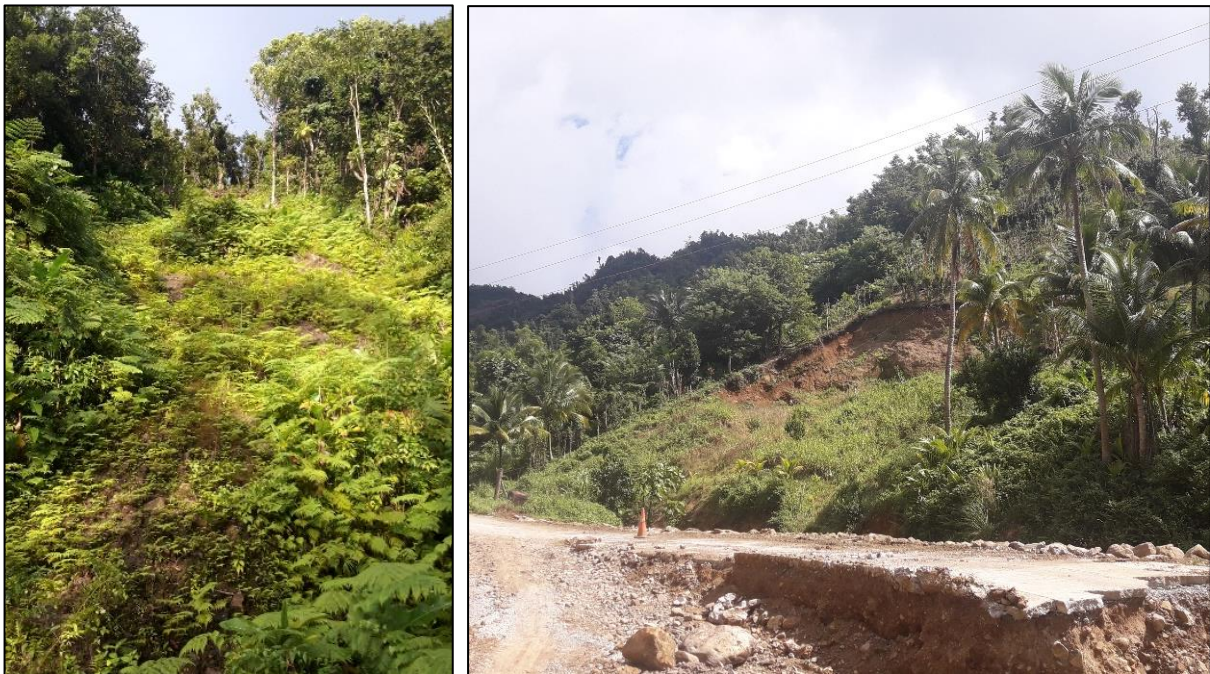
Figure 5.1. The state of the vegetation on two landslides in the Grand Bay catchment triggered by Hurricane Maria (photos taken by K. van 't Loo in November 2019).
