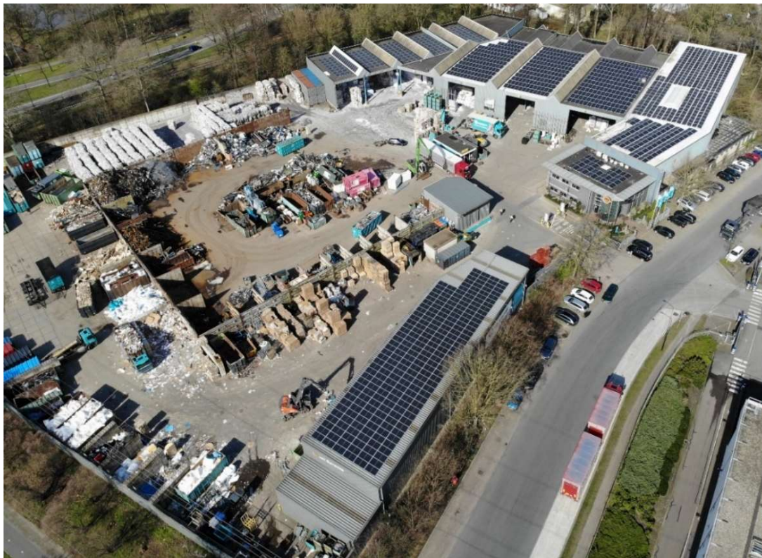
Figure 3-1 Current situation at Van Gerrevink
