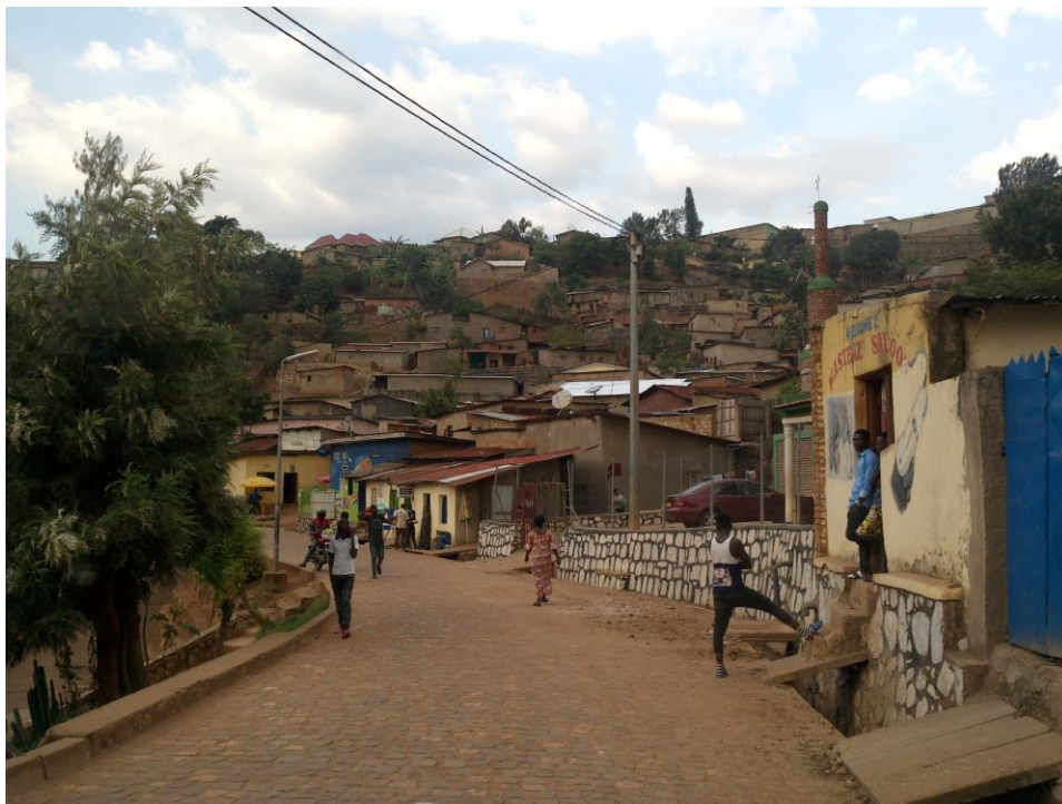
Figure I- 2 - unplanned settlements on the hillslope and paved road with drains on either sides of the road
