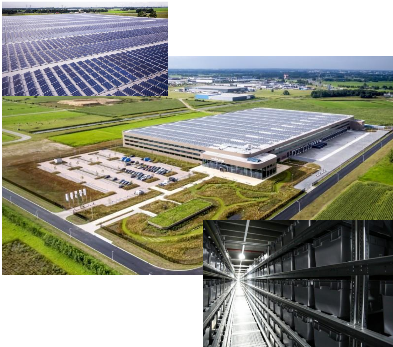
Figure 1.2 LSCZ, its solar panels and totes inside the OSR
