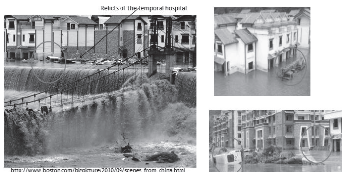
Figure 50. Damage by 2010 flood event
