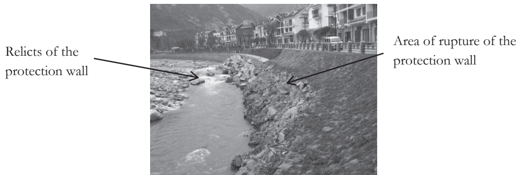
Figure 45. The wall protection broken by the Roa River
